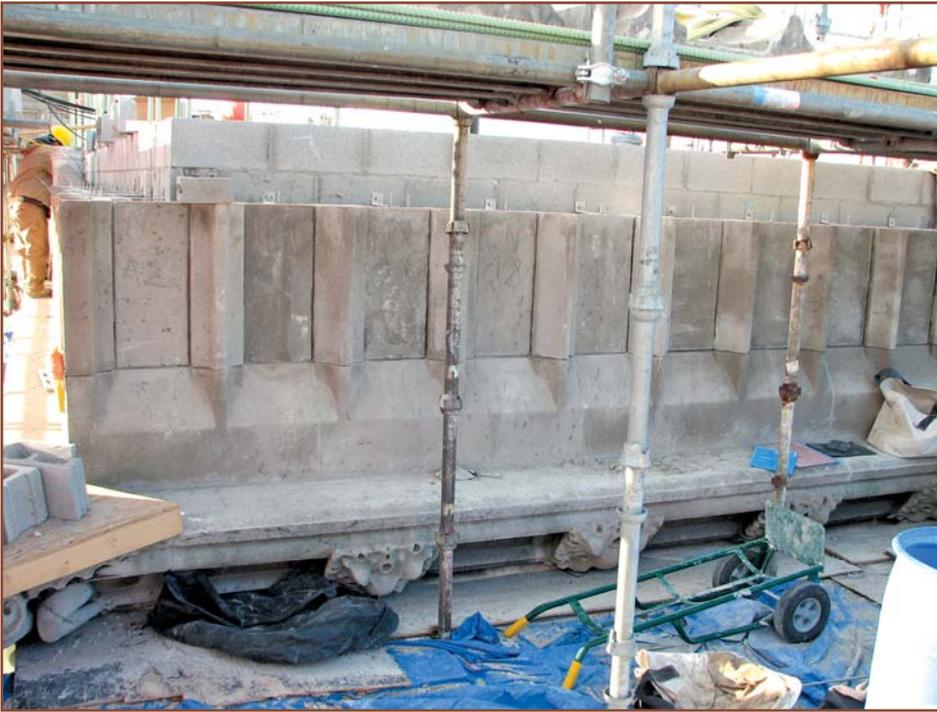
*Photo 7 – Reinstallation of cut/carved limestone cladding with stainless steel anchors.*
