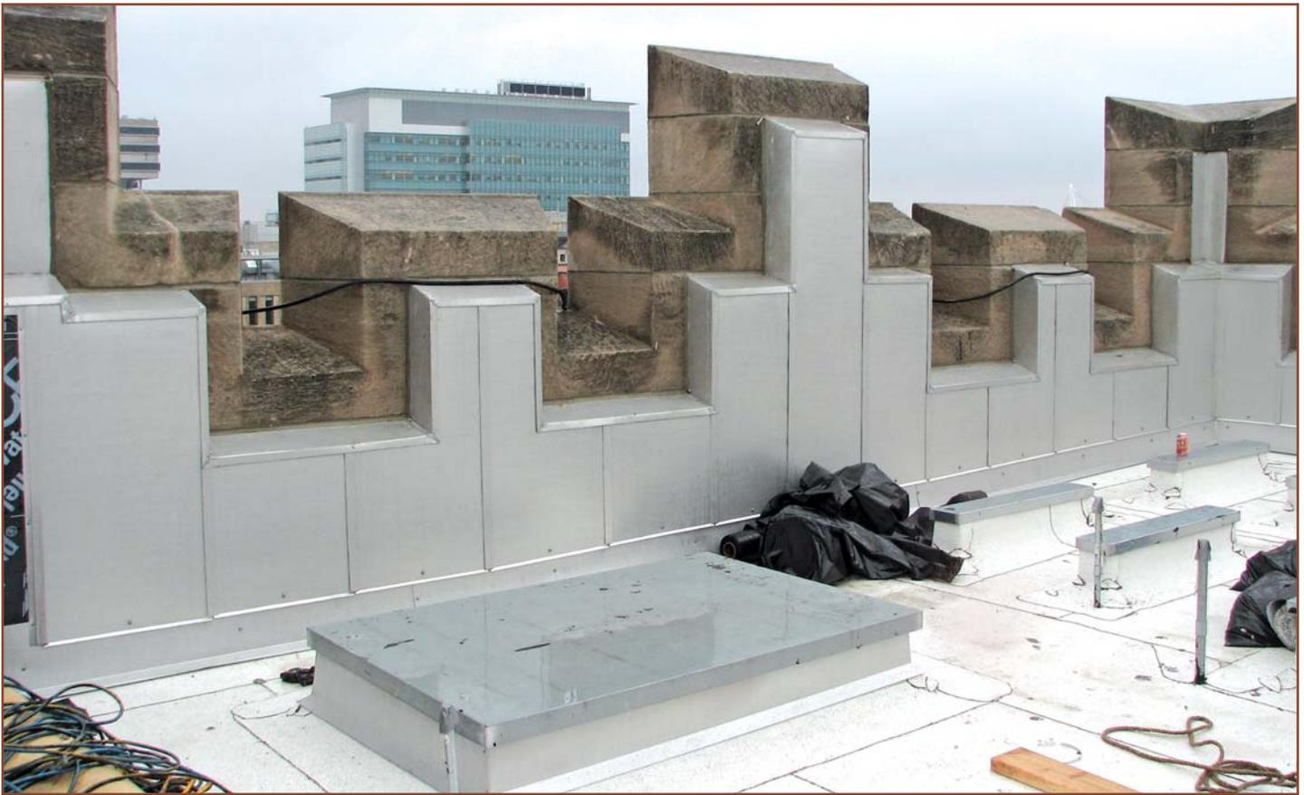
*Photo 10 – Fully completed parapet and new roof assembly.*
