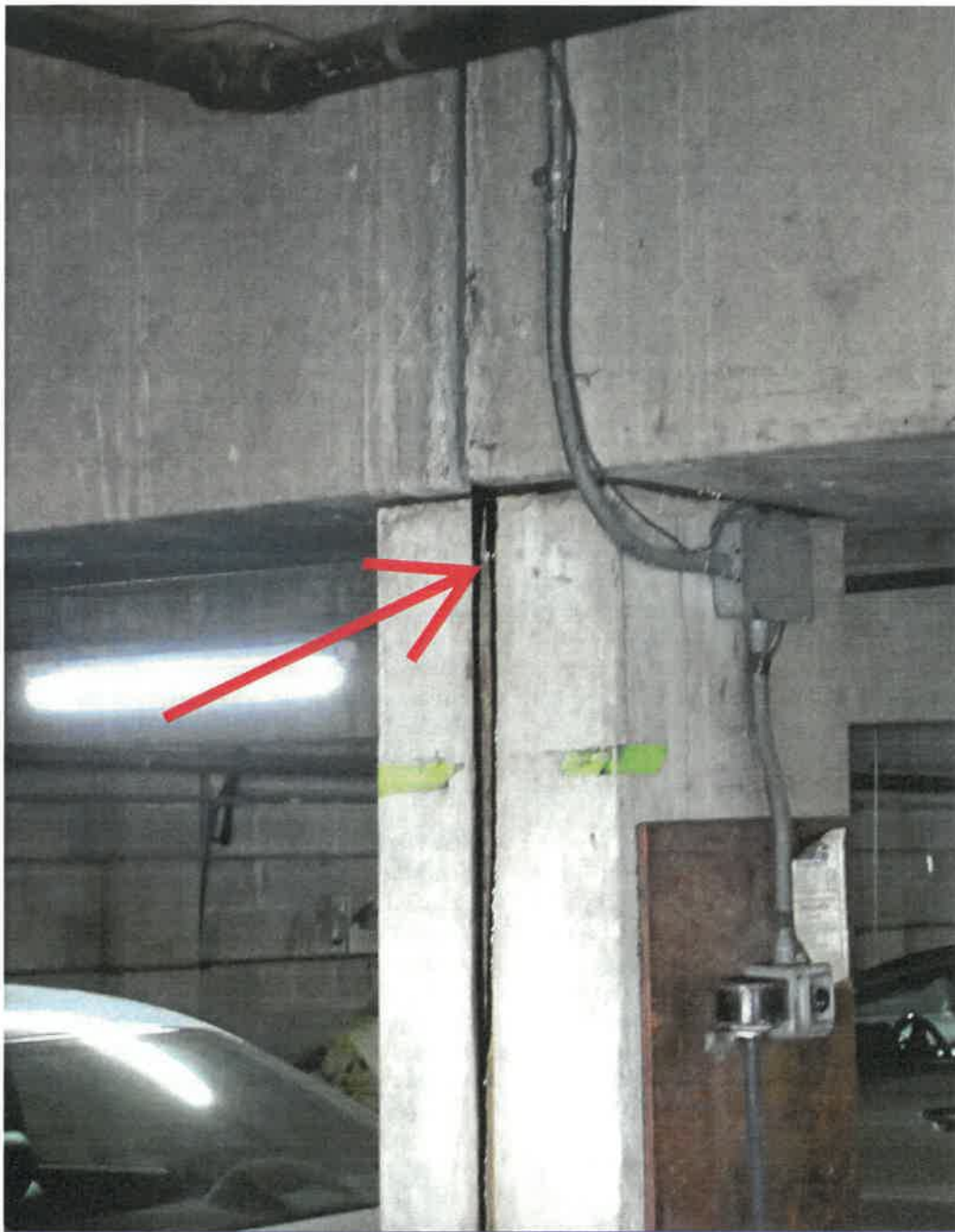
Figure 6. Polymer-gel migrating down through improperly predetailed substrate joint.
