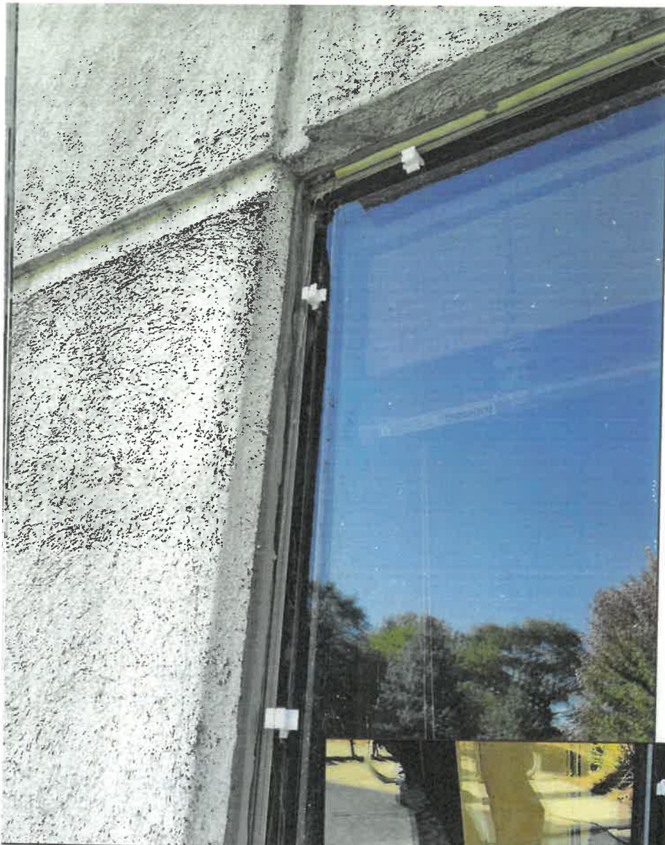
Figure 4. There was no evidence of existing weep holes, which would have provided drainage of water to the exterior. Photo courtesy of Inspec.
