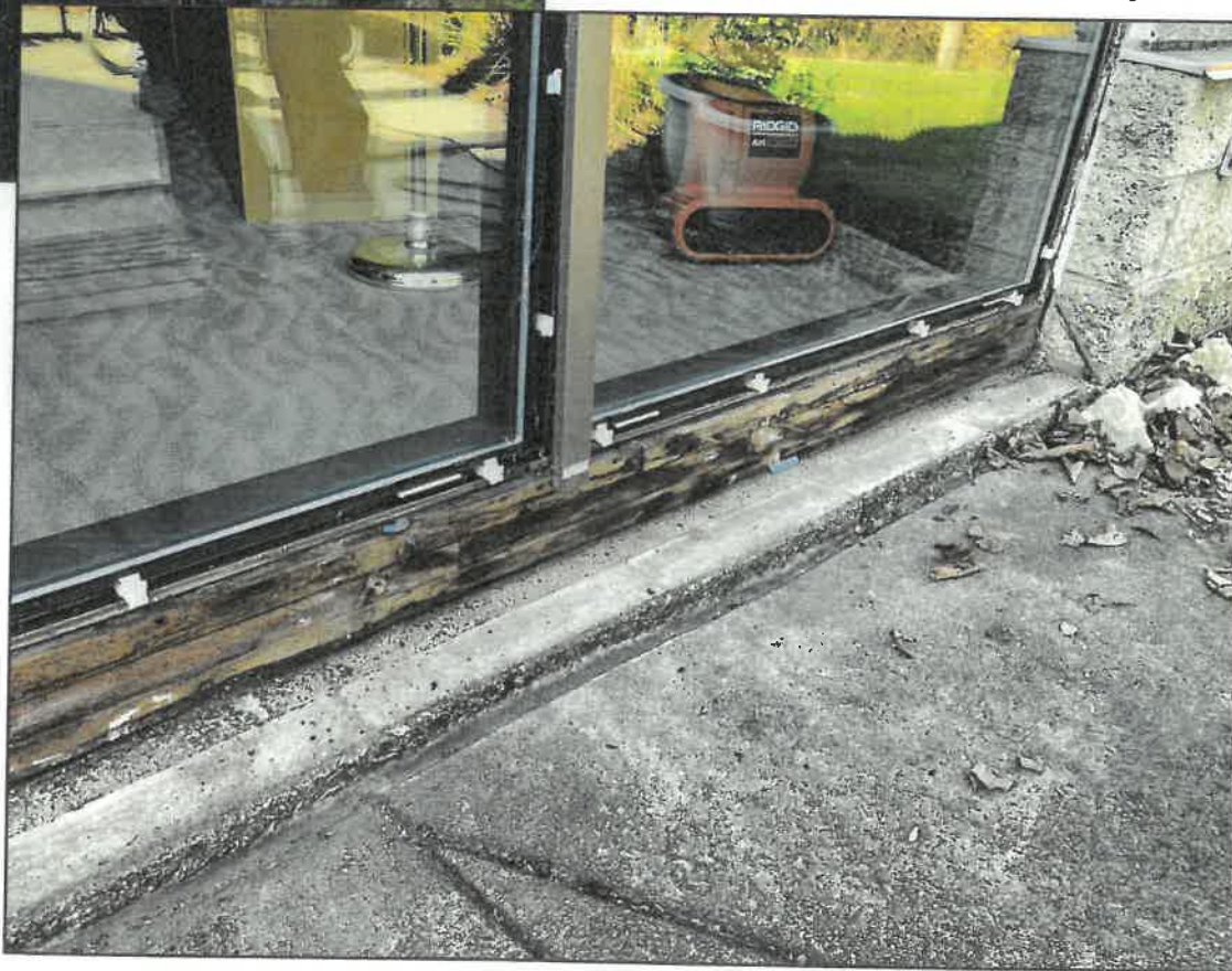
Figure 4. There was no evidence of existing weep holes, which would have provided drainage of water to the exterior. Photo courtesy of Inspec.
